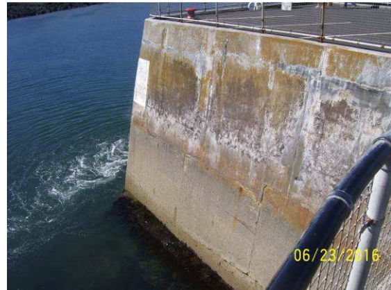
South East corner to stub 1701/C09
