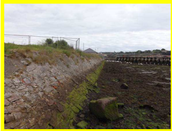
Masonry revetment 901c04 at northern end.
