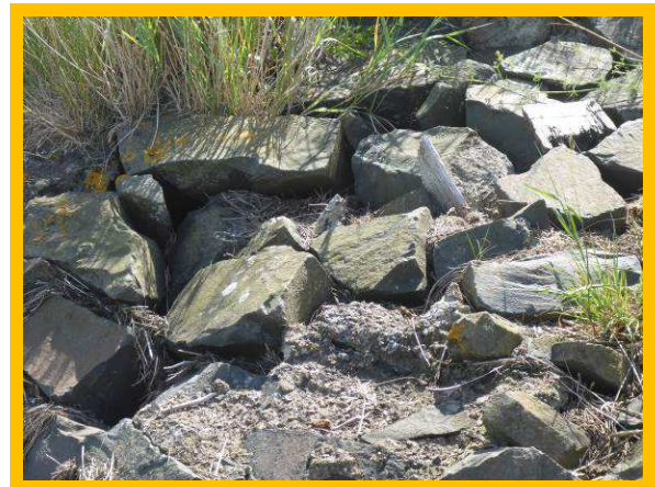
1401C98 – generally fair but locally poor stone-revetted embankment.
