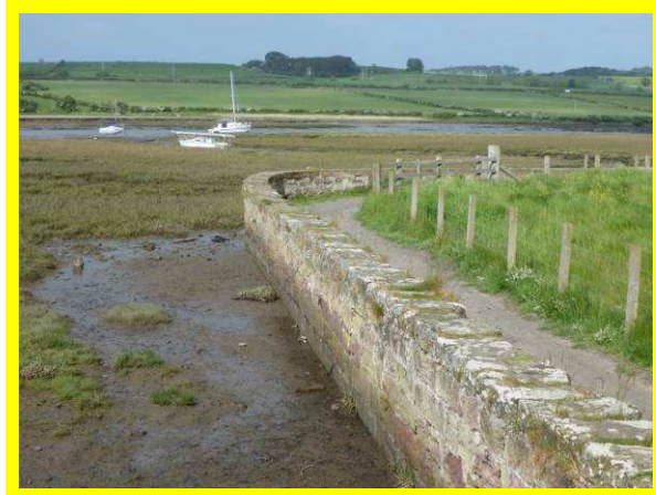
Masonry wall fronted by salt marsh (/2801C06)
