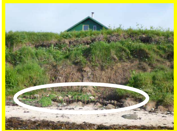
Local timber breastwork at toe of eroding cliffs (/2601C08)
