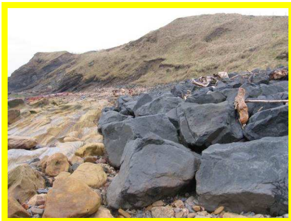
1001 c04/ 05 – low foreshore levels and erosion and slippage of coastal slope in 2006.
