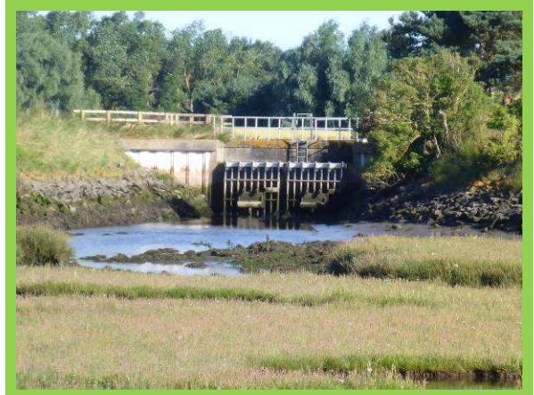
1401C16 – Good condition sluice at Ross Low channel
