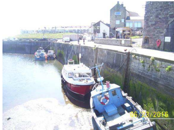
No signs of deterioration 1701/C13
