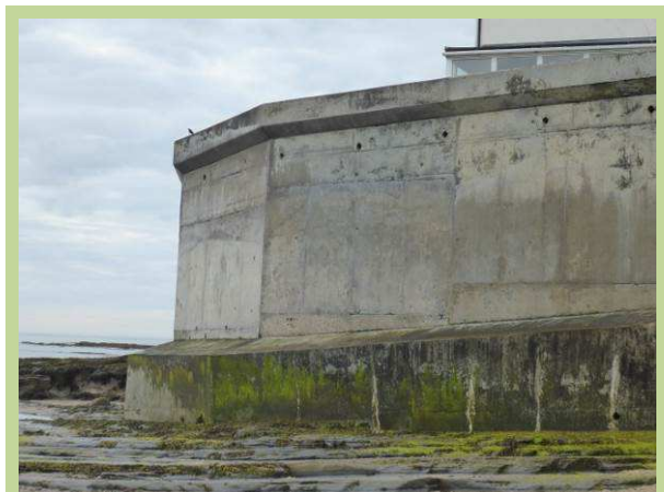
Substantial seawall in overall good condition (/3101C07)
