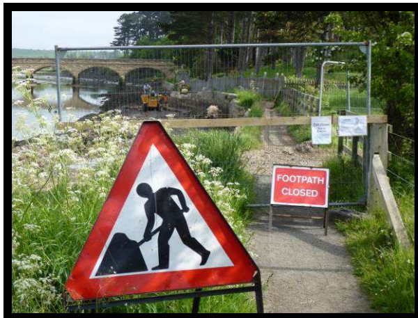
Footpath closure for repairs (/2801C10)
