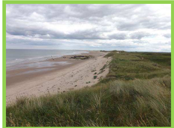
1201/ C02 – 2016 showing set back of frontage but higher beach levels and accumulation of sand to front face.
