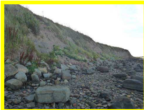
Eroding section of higher cliff (/4901c03).
