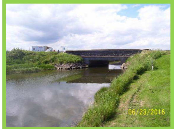
1701/C23 bridge to Annstaed Burn
