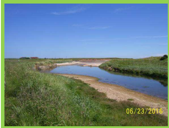
Minor areas of erosion and some areas of toe dune development to Annstaed Burn.
