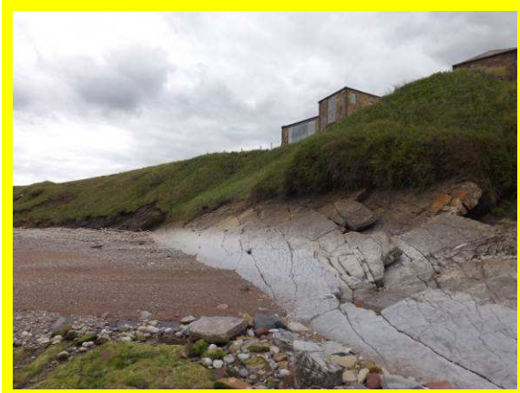
1101/c04 Sea House possibly constructed to rock with erosion of surface cover.
