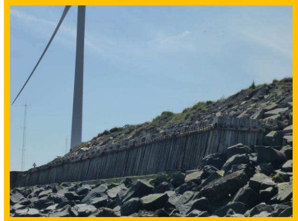
Composite defence with timber breastwork (/4001C03)
