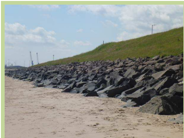
Rock revetment protecting former foundry site (/3901C05)
