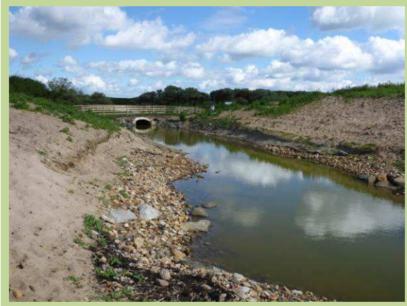
Landward view of newly 'daylighted' open channel section of outfall from Hauxley Nature Reserve (/3201C09)
