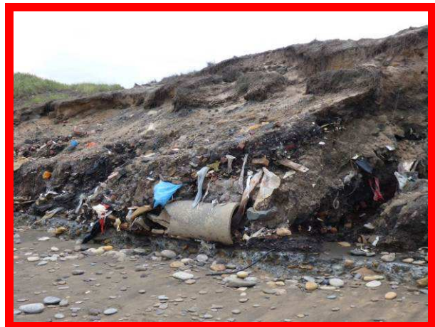
Actively eroding spoil cliff (/3401C05)
