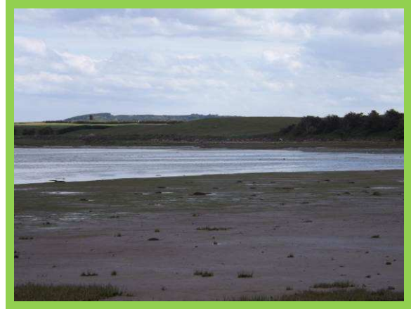
1401/ C24, Minor erosion to bank to rising land.
