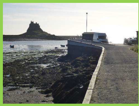
Improvement works to harbour pier (/4901c09)
