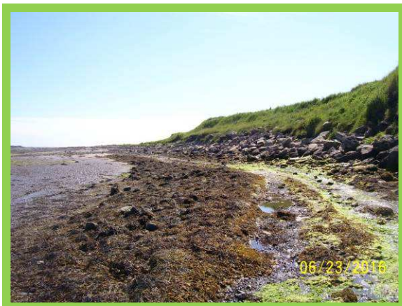
1701/C19 minor erosion above rock
