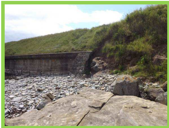
Outflanking of northern end of wall 1701/C54 - 2016
