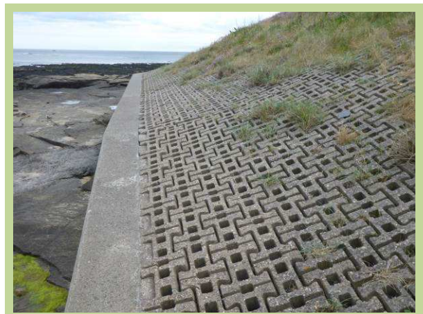
Low concrete wall and interlocking concrete unit revetment at Cresswell (/3201C19)
