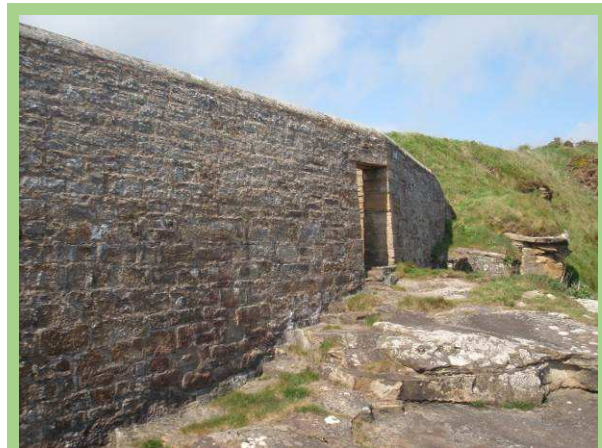
Masonry wall at The Bathing House in good condition (/2401C02)
