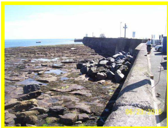
Rock armour wave reduction 1701/C06 – C07
