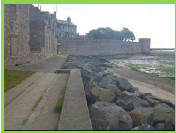
Rock revetment in good overall condition (/0801C04)
