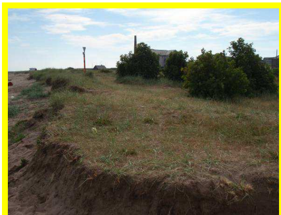
901c08 - erosion in 2012.
