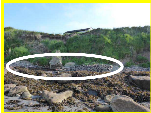
Local stone built wall at toe of eroding cliffs (/2601C08)
