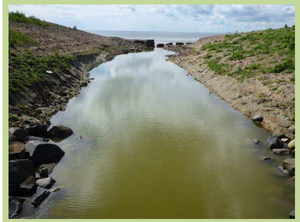
Seaward view of newly 'daylighted' open channel section of outfall from Hauxley Nature Reserve (/3201C09)
