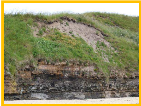
Slumping in cliffs at Greens' Haven (/0701C08)
