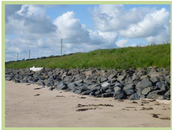
Wide rock revetment in good condition (/3201C03)
