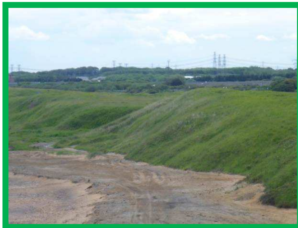
'Dormant' section of cliff protected by spoil beach (/3401C01)
