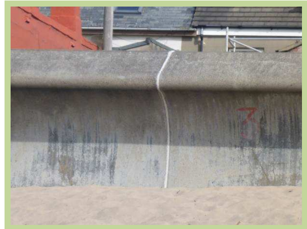
High beach levels and well-sealed joints in central sections of Newbiggin Bay (/3601C07)
