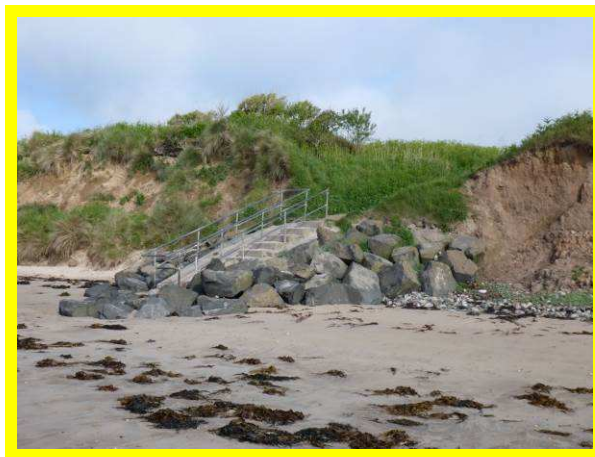
Rock armour around access steps in north of Foxtton Bay (/2601C09)
