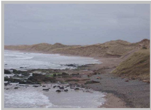
1201/ C02, C03 – 2006 showing recent erosion but dune system further forward than present day
