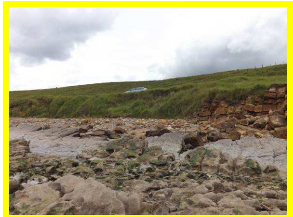
1101/c05 Critical section of frontage closest to road.
