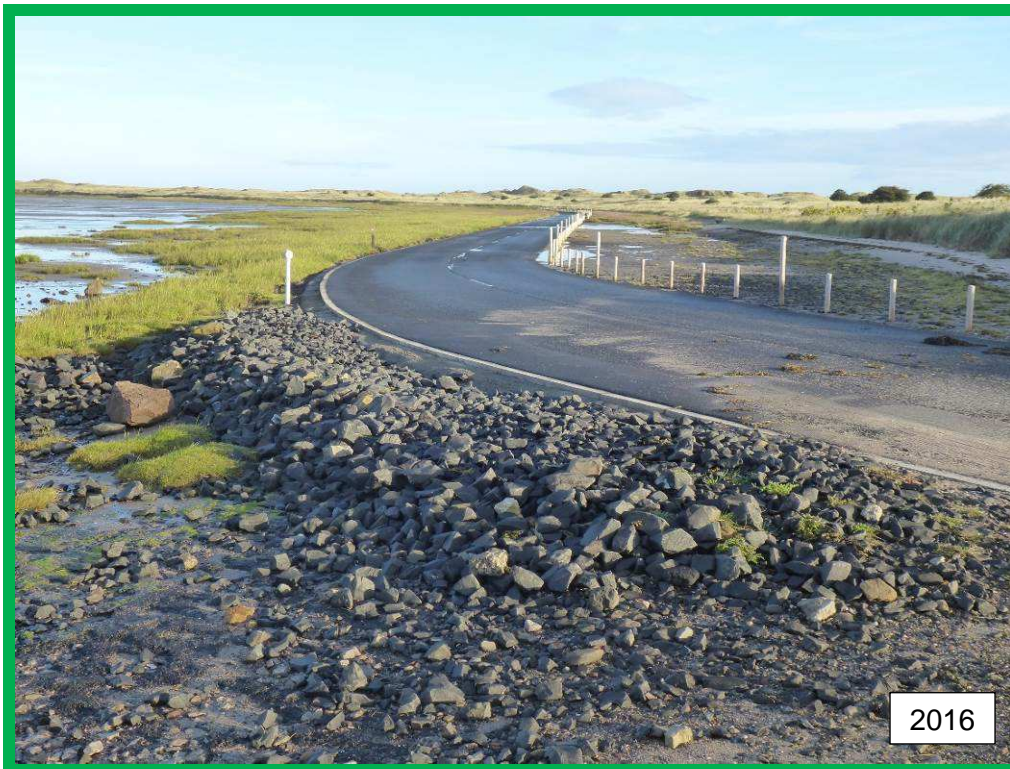
Repaired road surface and kerb at Chare Ends in 2016 (4901c01)
