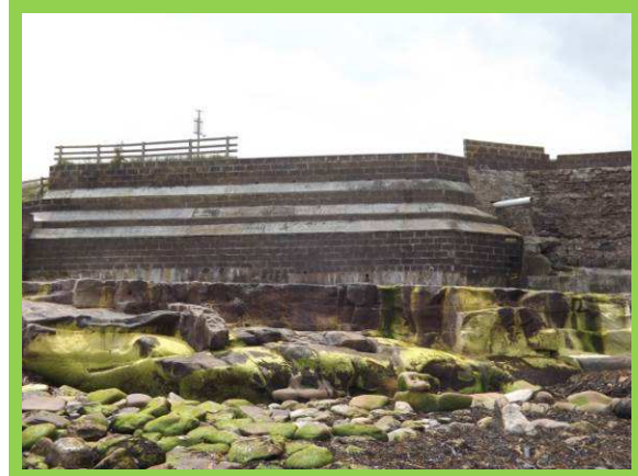
No significant damage 1701/C04 - 2016
