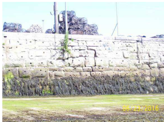
No signs of deterioration 1701/C14
