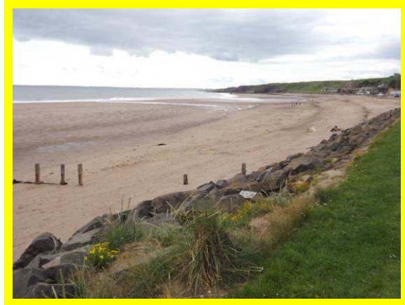
1001 c01 – showing no worsening of erosion at crest but also showing alignment in advance of natural beach shape.
