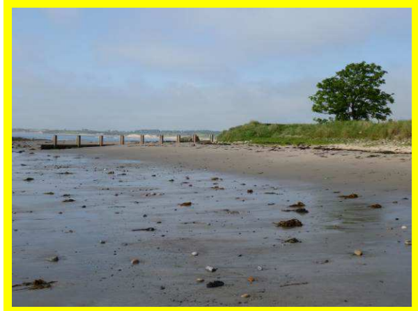
Isolated timber groyne (/2701C04)
