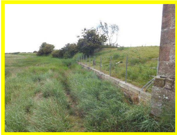
1401/C23 – local defence north of slipway.
