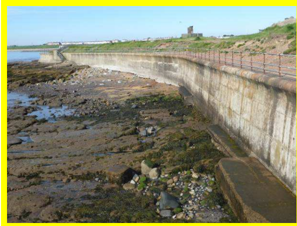
Church Point seawall in fair overall condition (/3601C12)
