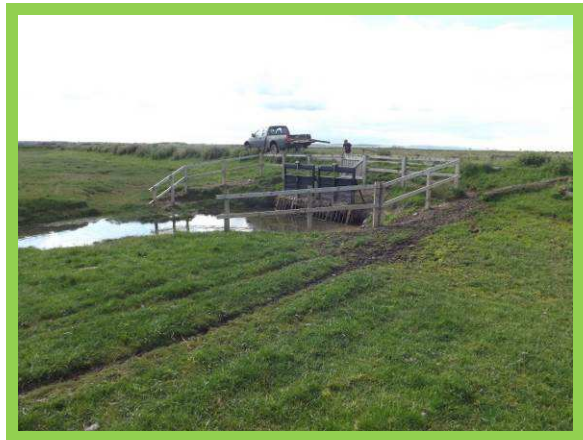
1401/ C31, Sluice to South Low. New fencing installed.
