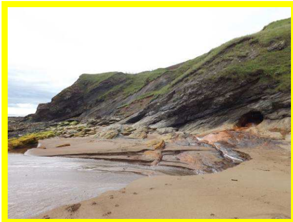
General slippage and erosion of lower coastal slope to 1001/ C05
