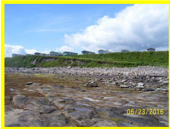
Erosion to access ramp 1701/ C22
