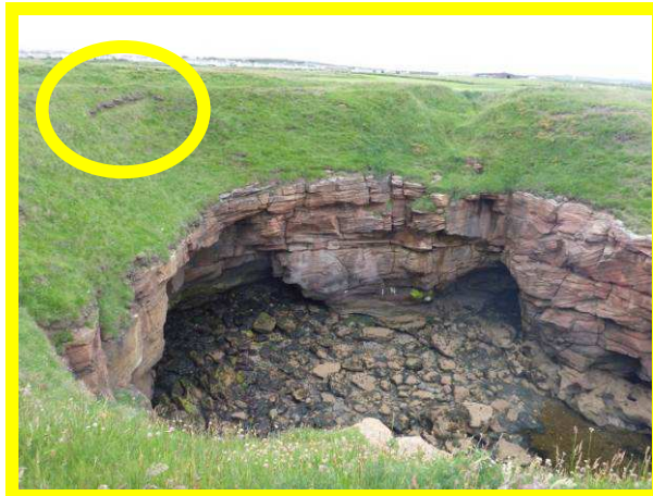
Localised slumping at Brotherston's Hole (/0701C01)
