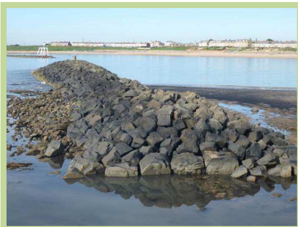
North breakwater in Newbiggin Bay in overall good condition (/3601C13)
