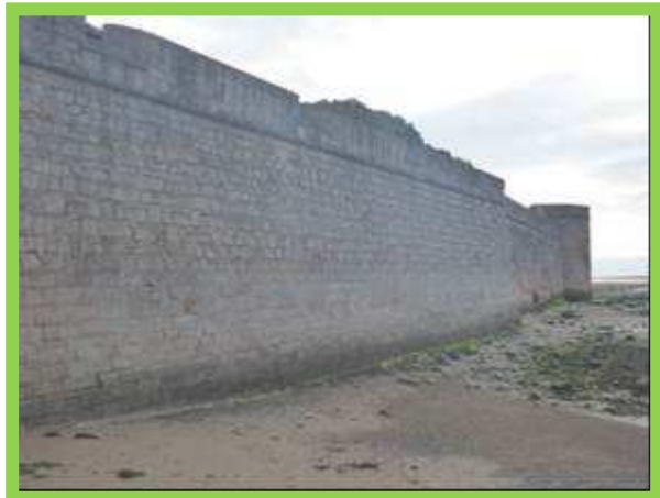
Berwick's historic town walls in good overall condition (/0801C06)
