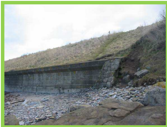
Outflanking of northern end of wall 1701/C54 - 2006
