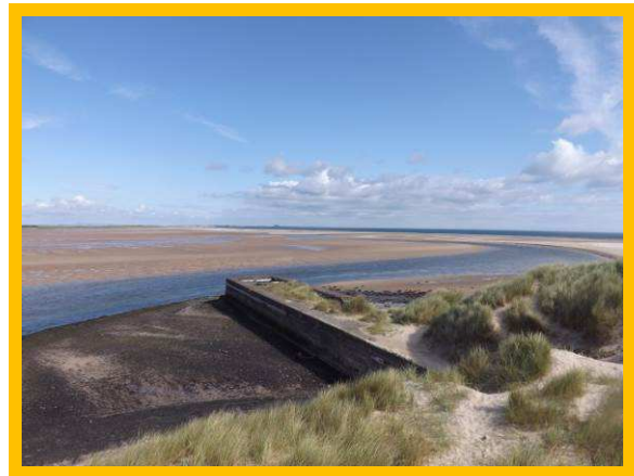
1501/C06 – south face and core of jetty
