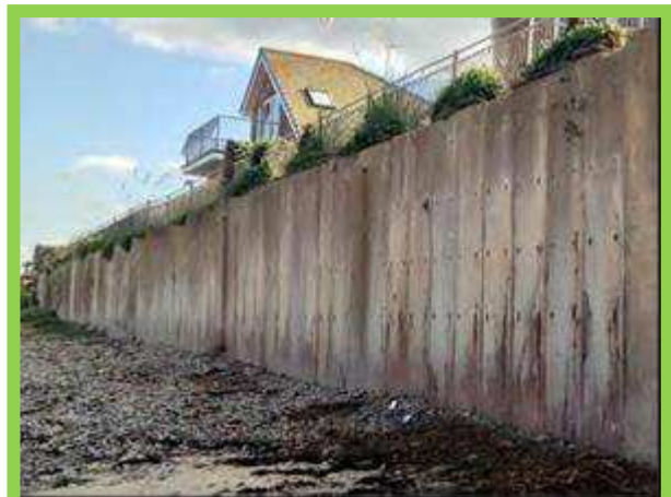
Good condition seawall (/1701C31)
