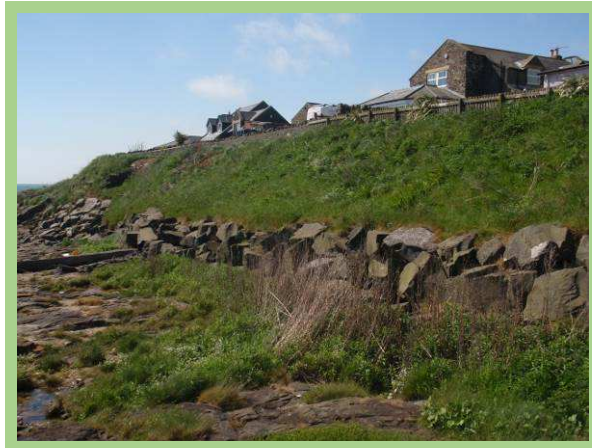
Inactive slopes with rock revetment at toe (/2201C13)
