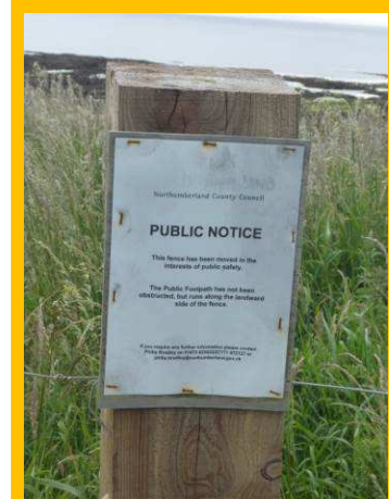
Relocation of fencing and footpath due to slumping cliffs along Magdalene Fields (/0701C12)
