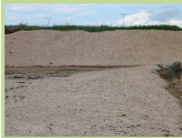
Stabilised, replenished and re-profiled dunes near Meggie's Burn (/4301C01)
