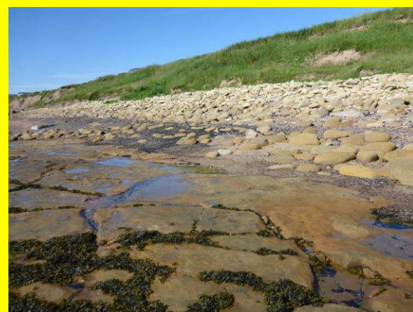
Slopes stabilised due to protection by sandstone boulder berm at toe (/3701C02)
