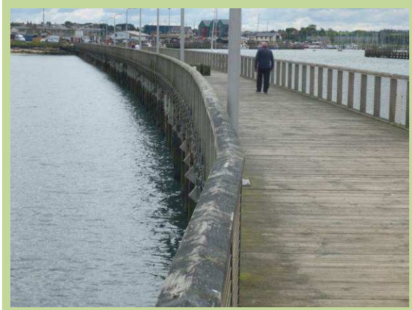
South Jetty in good overall condition (/3001C11)
