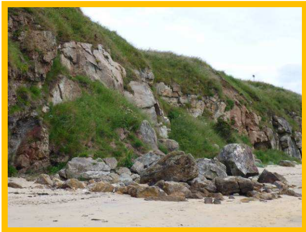
Rock fall in cliffs at Green's Haven (/0701C05)
