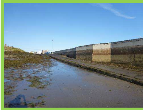
Improvement works to harbour pier (/4901c09)
