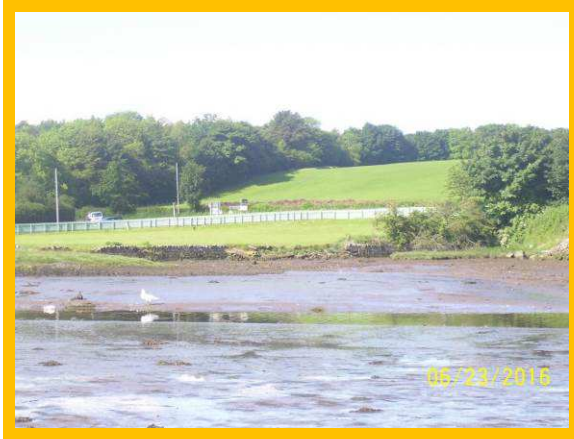
1501/C02 – poor condition of masonry wall
