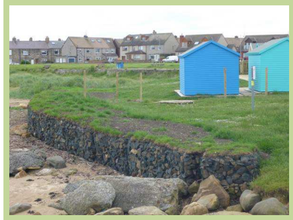
New gabions and beach huts (/3001C07)
