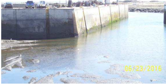
Inner face of the Inner Pier 1701/C10
