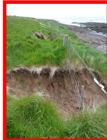
Coastal slope erosion at Newton Point headland (/2001C01)
