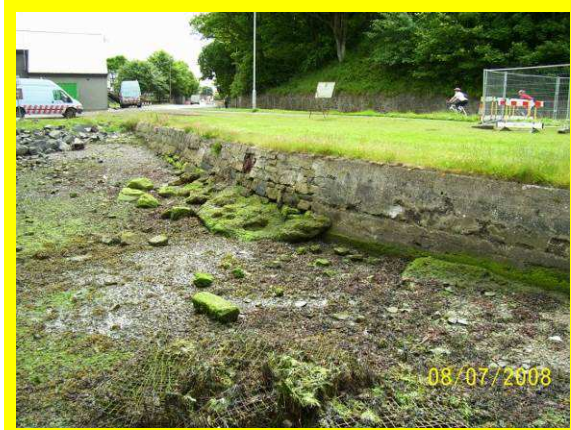
901c06 in 2008 showing toe level and condition of masonry.
