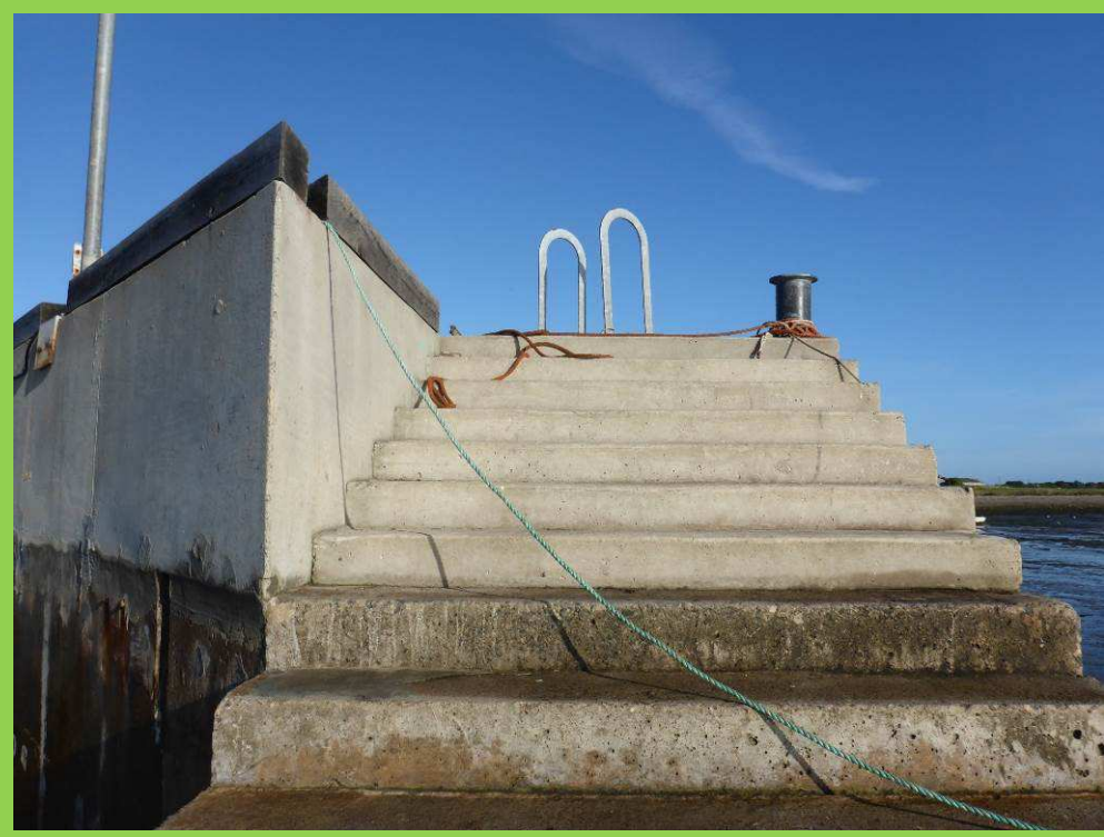
Improvement works to harbour pier (/4901c09)
