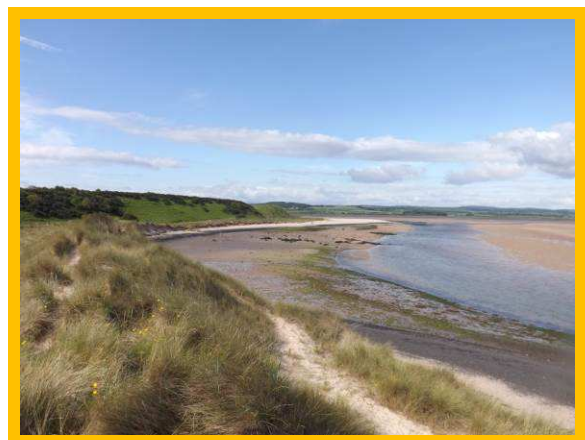
1501/C06 – 2016 major area of erosion to south of jetty
