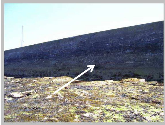
Developing abrasion hole 1701/C07 2010
