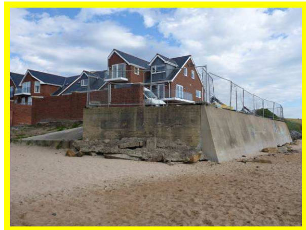
Existing sea wall protecting new properties (/4201C04)
