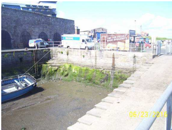
No signs of deterioration 1701/C12
