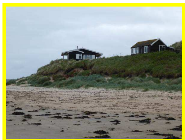
Previous dune damage followed by recovery at Newton Haven (/2001C03)
