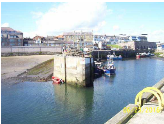
No signs of undermining 1701/C14
