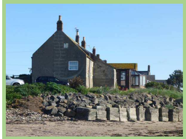
Stacked concrete blocks (original scheme) and rock revetment (emergency scheme) at southern end of Boulmer village (/2601C05)
