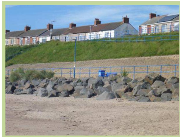
High beach levels fronting rock revetment (/3601C08)
