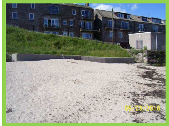
1701/c16 Good condition, no sign of undermining.
