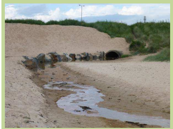
Rock armourstone placed in 2016 to train course of Meggie's Burn away from dune toe (/4301C01)
