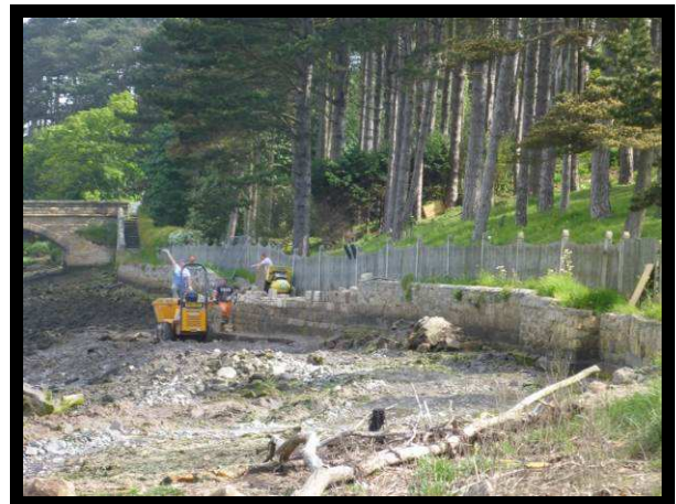
Repair of masonry riverbank wall (/2801C10)
