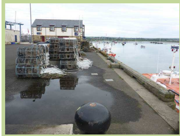
Quay wall in good overall condition (/3001C05)
