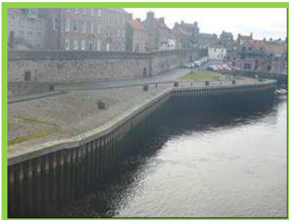
Steel sheet piled quay walls in good overall condition (/0801C03)
