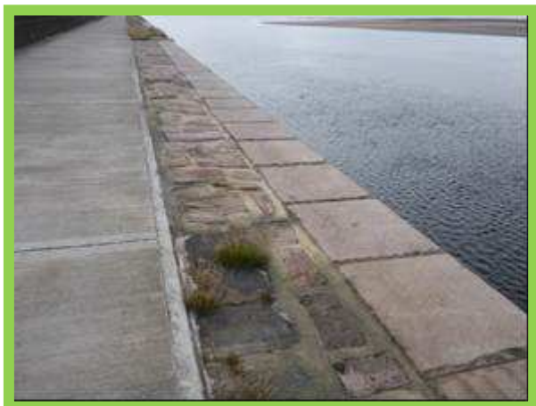
Repairs to deck and southern face of Berwick Pier (/0701C15)
