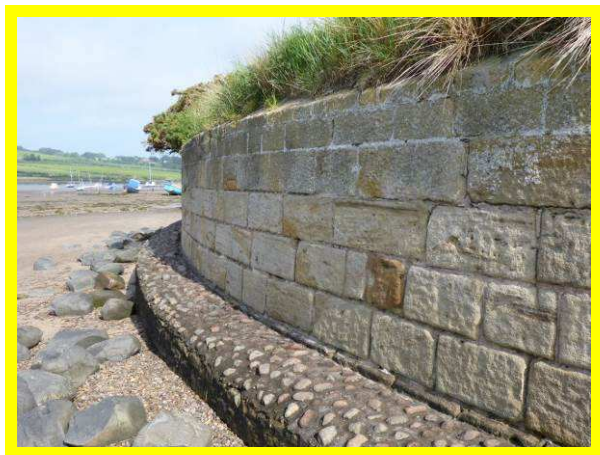
Masonry wall with concrete and cobble toe apron (/2801C02)
