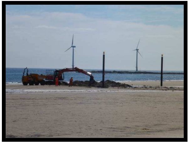
Repair works to outfall on foreshore (/3901C04)
