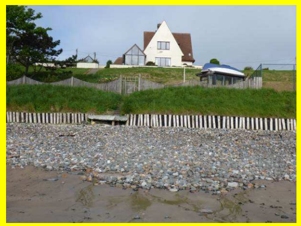
Timber breastwork fronting property (/2701C02)
