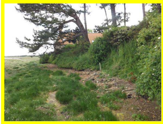
1401/C23 – local timber defence.
