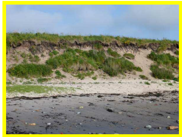
Local slumping to dunes around Seaton Point (/2601C07)
