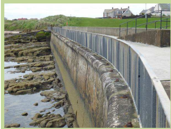
Seawall in good condition despite rust-staining (/3101C05)
