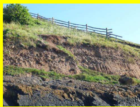
Slumps in cliff below castle east of erosion matting (/4901c12).
